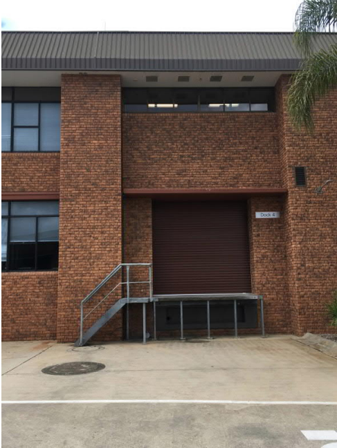
Figure 3.4.3 View of existing Dock 4 on printery - external north wall. Existing dock and dock leveller to be relocated to this existing dock location. Façade not visible from Zouch road,
