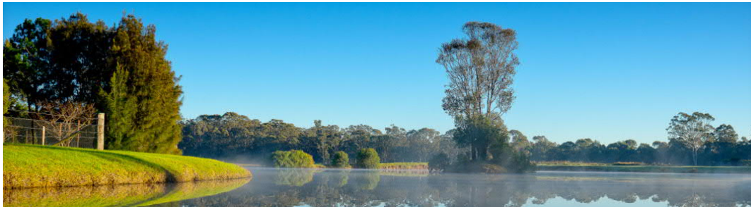
Figure 7.1.2 View looking west over large dam
