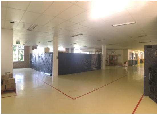
Figure 3.4.5 View of existing printery pre-production area. This area to include small modifications for additional offices for the AVS Department. Please refer to ANNEXURE A – ARCHITECTURAL DRAWINGS .
