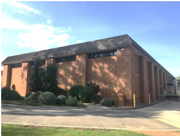
Figure 3.4.2 View of existing printery - external north east/north west walls. Existing windows to audio/video studio will be replaced with cladding to match existing finishes. Existing loading dock and dock leveller at Dock 3 will be relocated further west on the northern façade to Dock 4. New AC packaged unit installed in existing dock area. Not visible from Zouch road.
